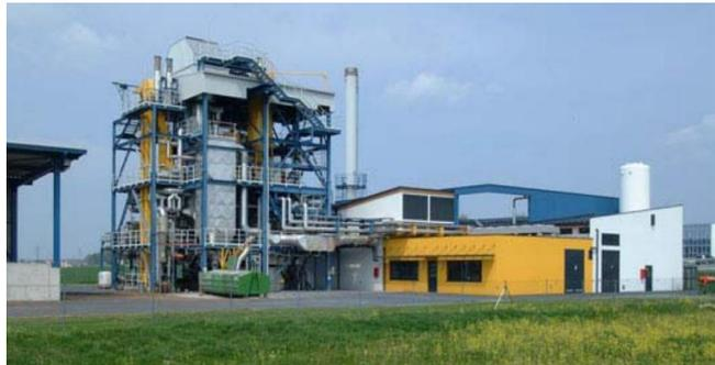
The plant achieves an electrical production of 2 MW from 8 MW of input biomass, through a biomass gasifier coupled with an Internal Combustion (IC) gas engine with an electrical efficiency of 25% and a heat efficiency of almost 50%. The gasification plant produces 4.5 MW of heat for the local district heating network.<sup>6</sup>
